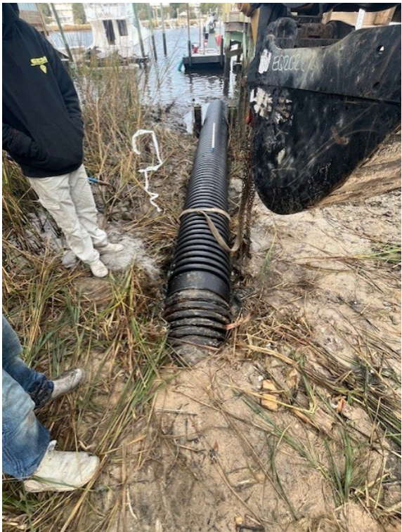
The outfall pipe at Sandpiper Lane has been replaced.
