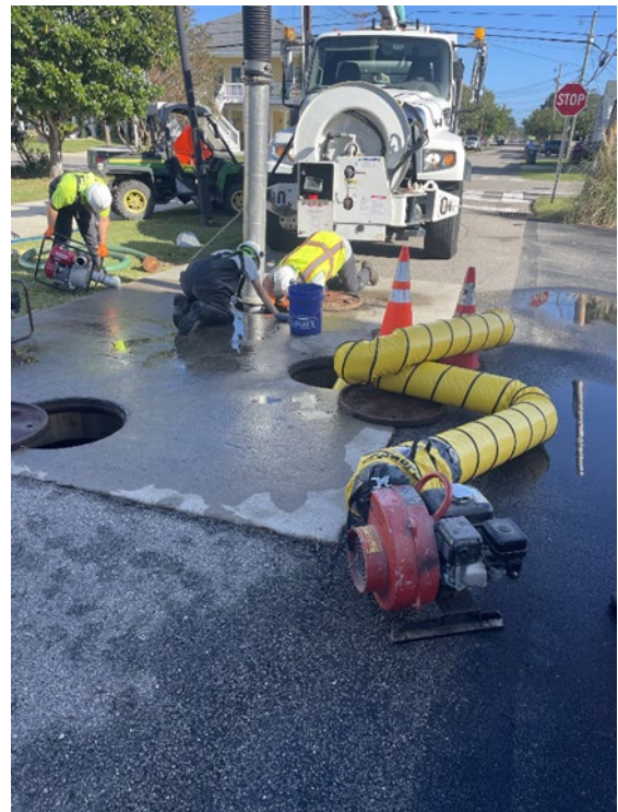
Stormwater crews clean out the sediment vault on Atlanta Ave.
