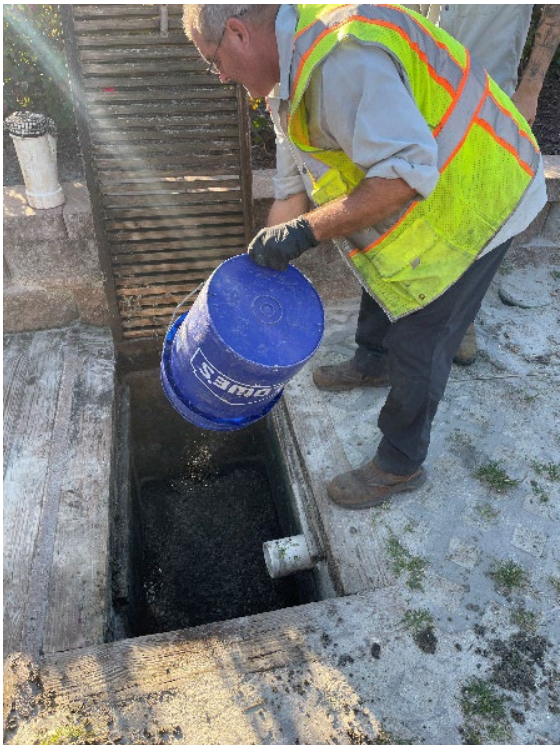
Stormwater crews replenish shower BMPs with fresh 57 stone
