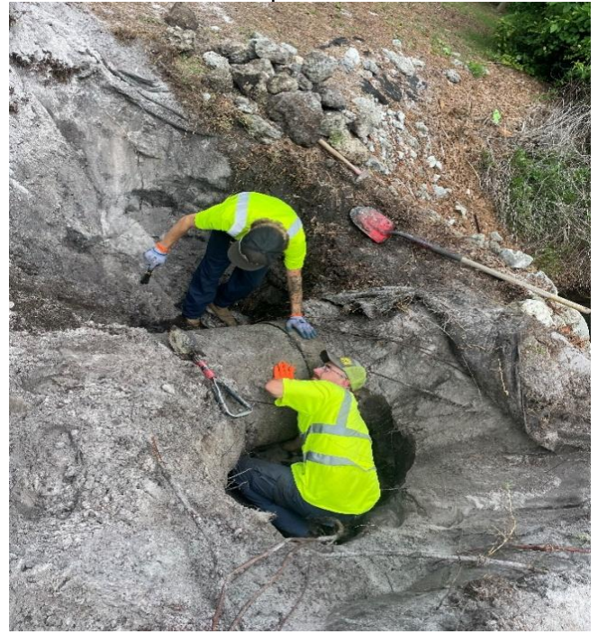
Stormwater department repaired sinkhole at the Town Hall pond/Civil War Park.
