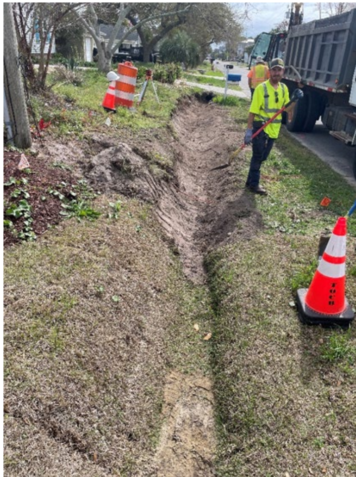
Stormwater crews re-establish ditch on the 500 block of Greenville Ave.
