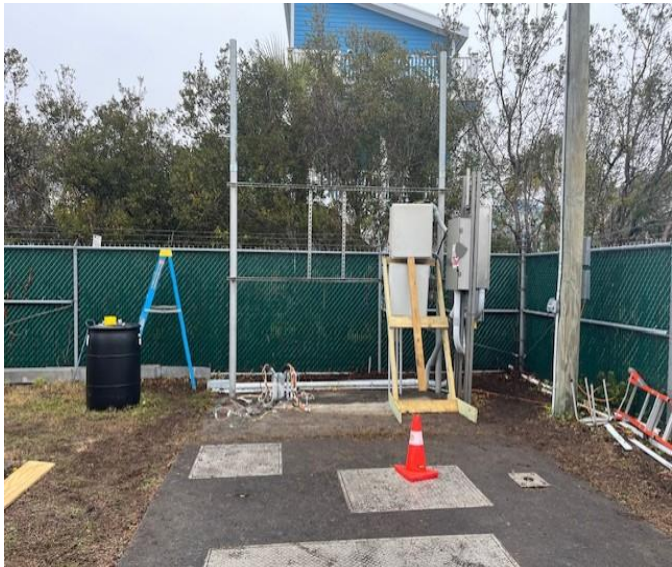
Elevating and replacement of theTexas stormwater pump control panel has started
