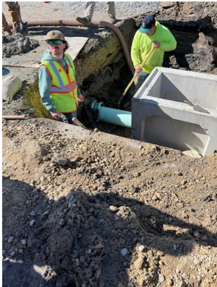
Contracted crews repair drain field at end of Delaware Ave.
